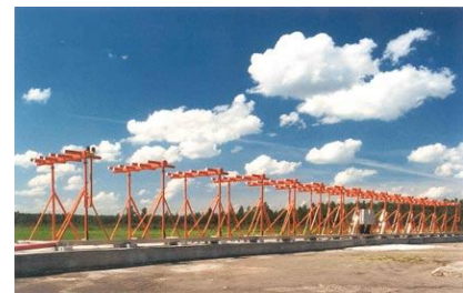
Struktur ground station antenna LOC
